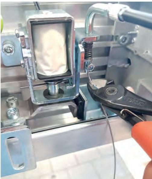
Cut the excess steel cable from the release anchor.
